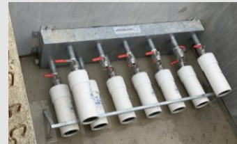
SKID PIPE for gravity drainage of remote pits, approx. 200 L/min
