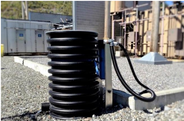
Petro Barrier Pumped PTB 24 outside the retention area, connected to a pump to filter the overflow from the remote pit - NATIONAL GRID
