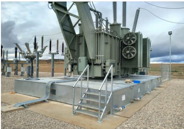
Modular Fire-Resistant Retention Tank ERT-MODULO 5 with access stairs and PETRO PIT filtration cartridges - REPSOL
