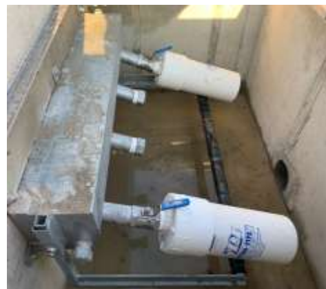
PETROPIPE PI-616-M2 alone or mounted on SANERGRID SKID 1x4 PETRO PIPE to drain by gravitation the transformer oil containment bund or concrete pit without risk of water contamination – EDF, CONEDISON or EXELON Group
