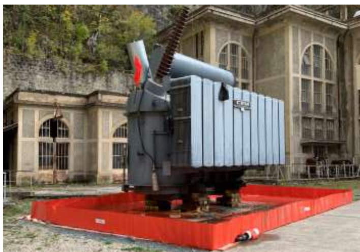
Flexible Storage Tank TRFLEX-ECO+ for temporary outdoor storage equipped with 2 SPI PETRO-PIPE PI616-M2 filters - EDF
