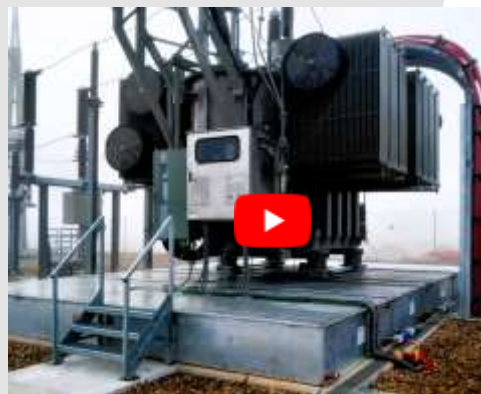
Power Transformer on SANERGRID TRT-MODULO 4 oil retention tanks equipped with SPI PIT416 drainage water drainage cartridges
