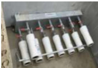
PETRO PIPE PI-616-M2 in SKID for gravity drainage of offset pits, approx. 200 L/min
