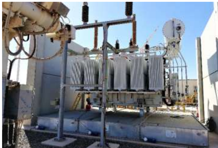
TRT-MODULO 3 Tank equipped with an EXTICOV LHD fire-resistant cover and PETRO PIT SPI filtration cartridge – NATURGY, IBERDROLA, SCHNEIDER, SNCF...
