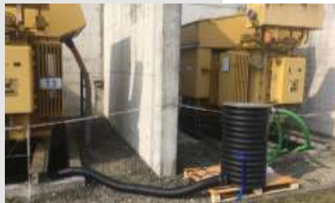
Power transformer concrete bund equipped with automatic sump pump and PETRO BARRIER™ filtration system
