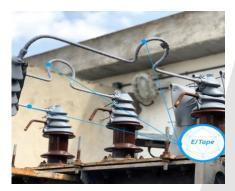
The 2 mm thick self-fusing silicone tape forms a custom insulating barrier and provides a 35 kV phase-to-ground insulation rating with a single layer, and up to 50 kV with a double layer. This tape is not recommended for use on highly irregular surfaces but is better suited for smooth or slightly contoured areas. For more complex geometries, other Midsun® solutions such as E/COVER or E/PLAQUE are recommended, or FUSE (documentation available upon request).
